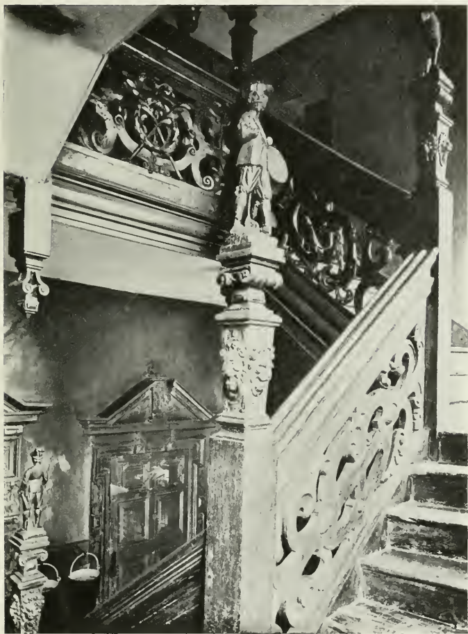
172. Staircase, Cromwell House, Highgate.
